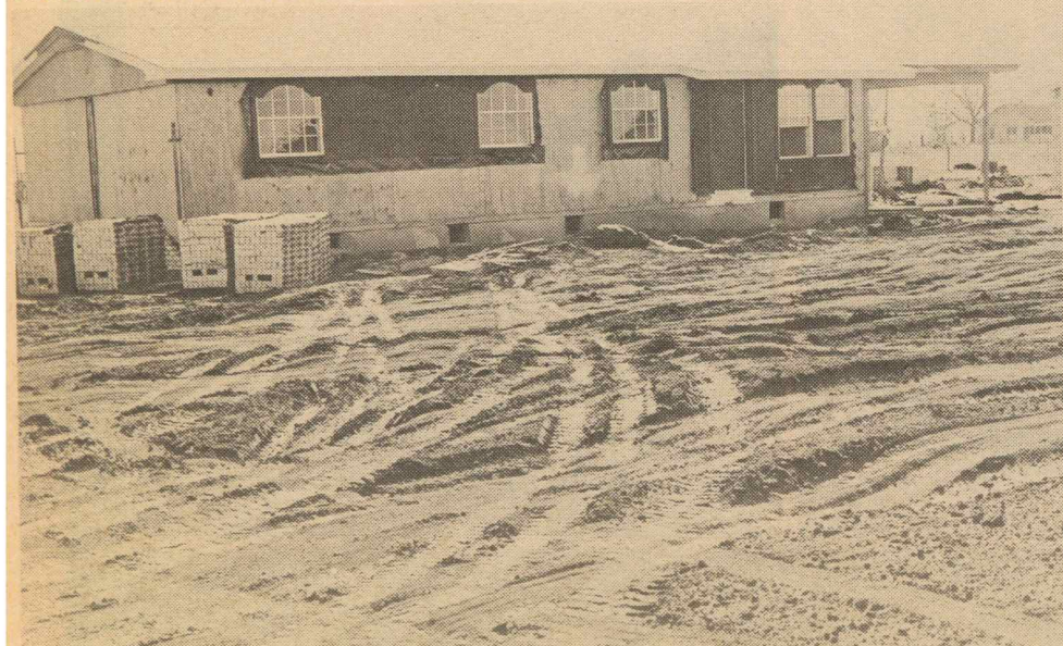
Full house on site, ready for brickwork.
