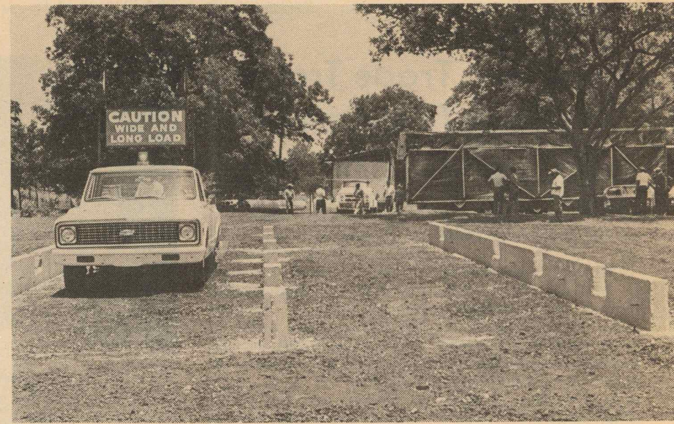
Sections moved toward waiting foundations.
