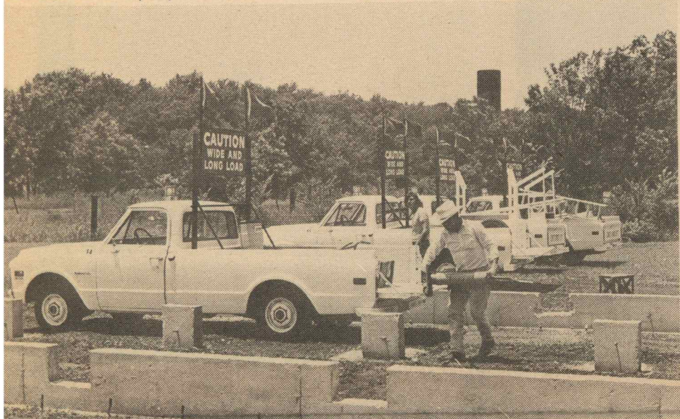
Jacks unloaded to receive house.
